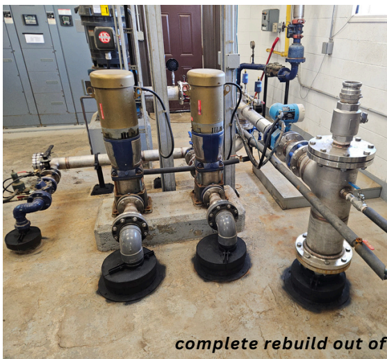
Distribution pumps feeding header
