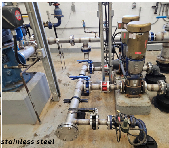
header into main trunk line
