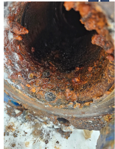
the inside of the original ductile iron piping
