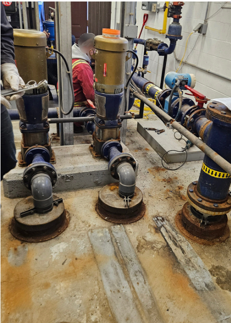
Distribution pumps feeding header
