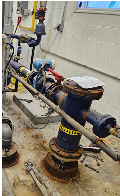
header into main trunk line
